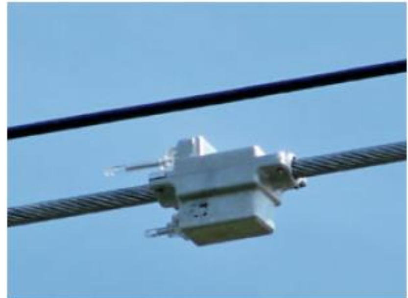
Monitors for dynamic line rating (DLR)
